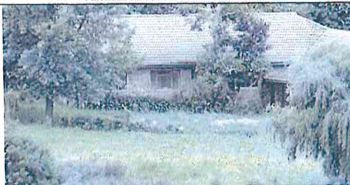
Derelict Farm House
