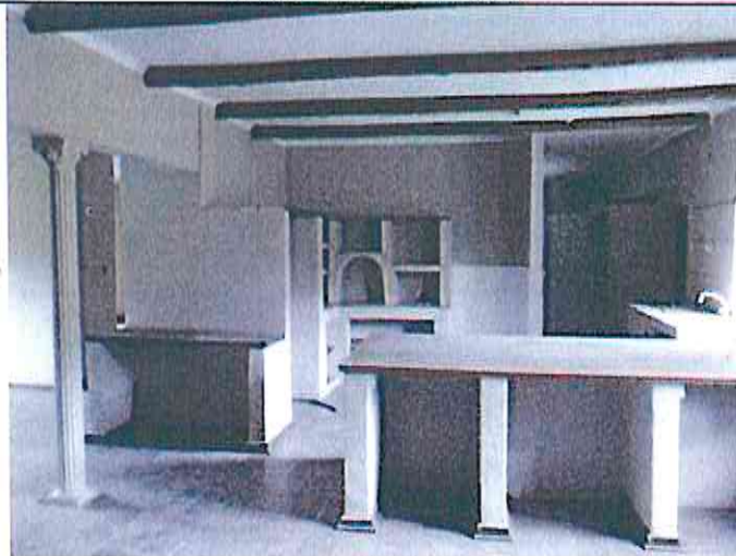
Derelict Farm House
