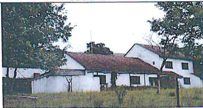
Derelict Farm House
